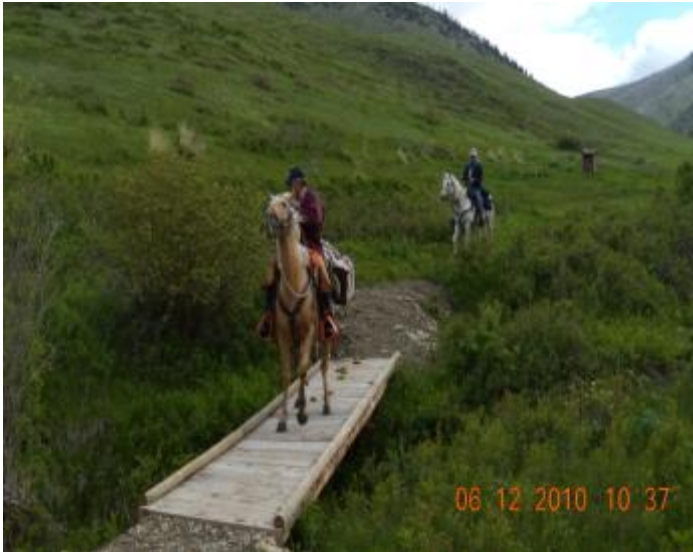
Bob and LeAnn crossing the bridge we built last year
