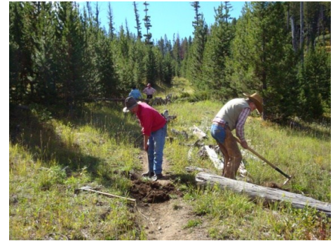
1 Installing a water bar at Bridger Bowl
