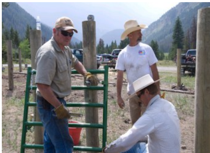
Gates are installed by Don Drake, Ed Long and Michael Harney.
