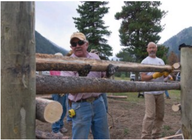
Mike Haugen and Ed Long put a rail in place.
