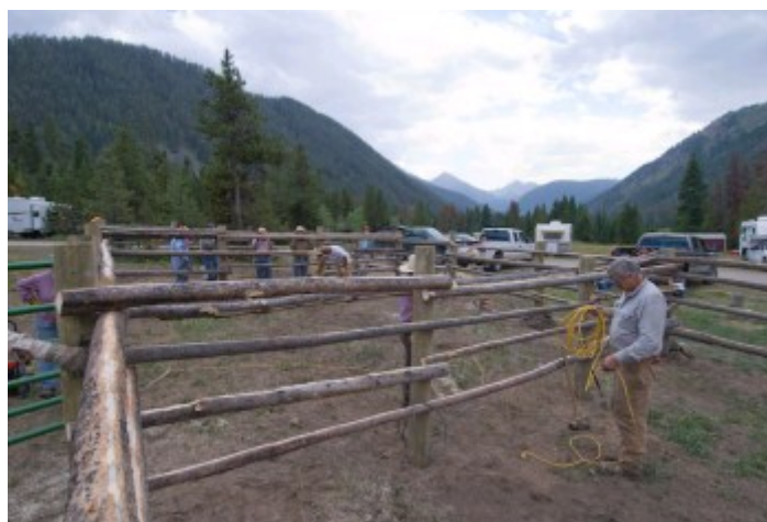
It's a wrap! Dan Marsh wraps an electrical cord as the project is completed.
